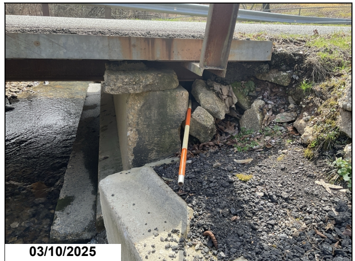
Bent 1 left side, 5' void behind abutment.
