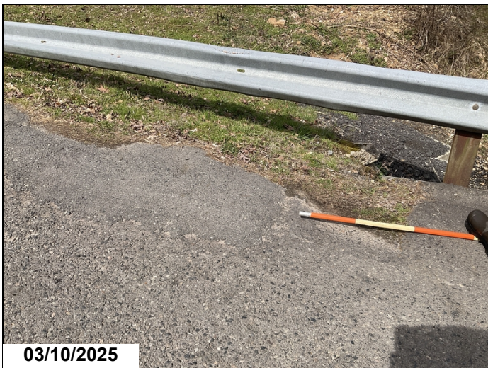
Bent 1, right side, up to 5' void behind abutment causing approach roadway to settle.
