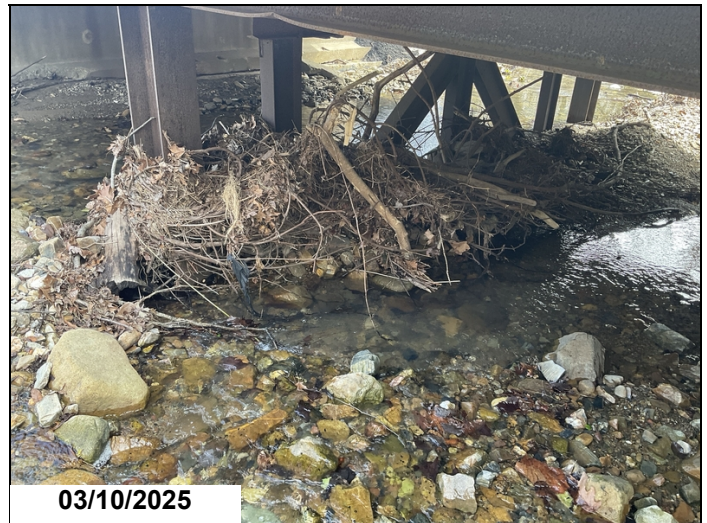
Drift and debris has accumulated at bent 2.
