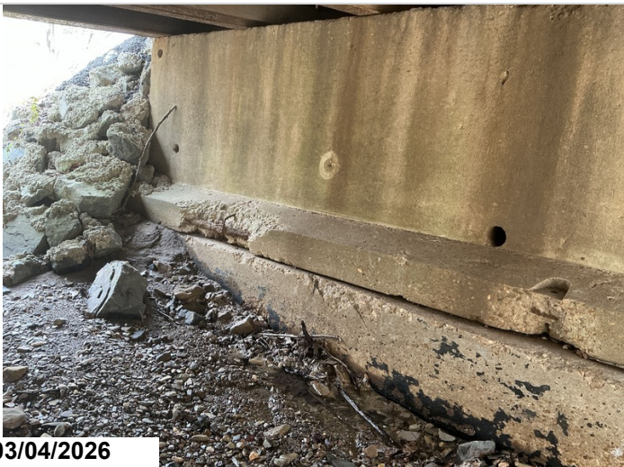
Bent 3 footing has a couple spalls with exposed rebar.
