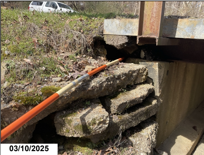
Bent 1, right side: up to 2' void behind abutment.
