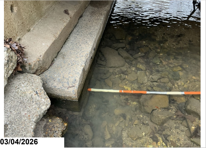
Bent 1 downstream footing is undermined up to 2'.
