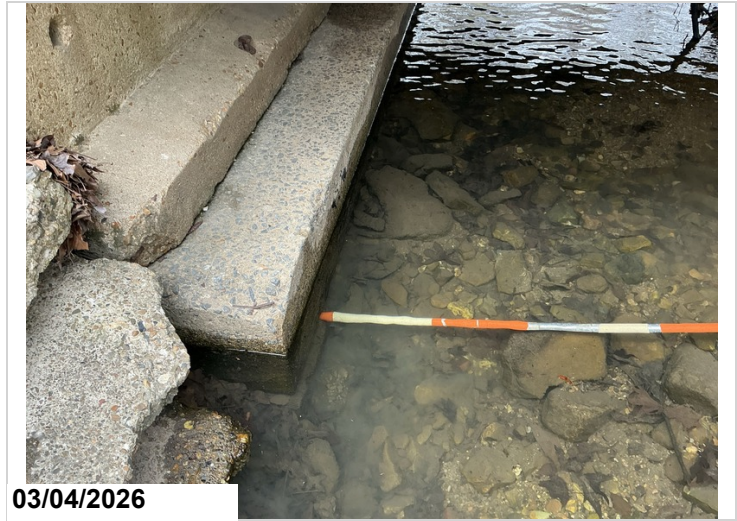
Bent 1 downstream footing is undermined up to 2'.
