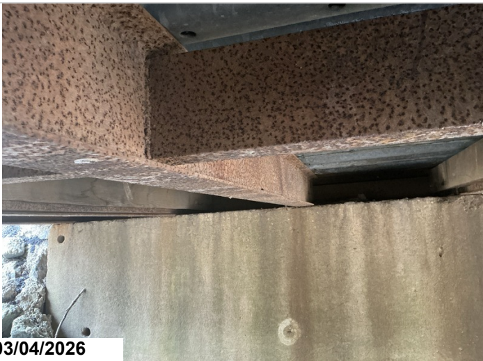
Span 2 girder 3: girder has active corrosion with moderate pitting. All girders in both spans are in similar condition.
