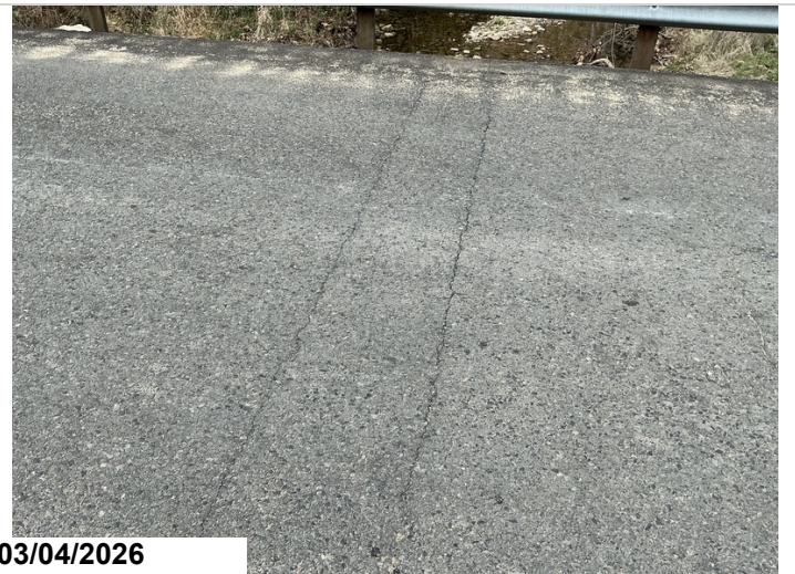
Transverse cracks in the asphalt wearing surface.
