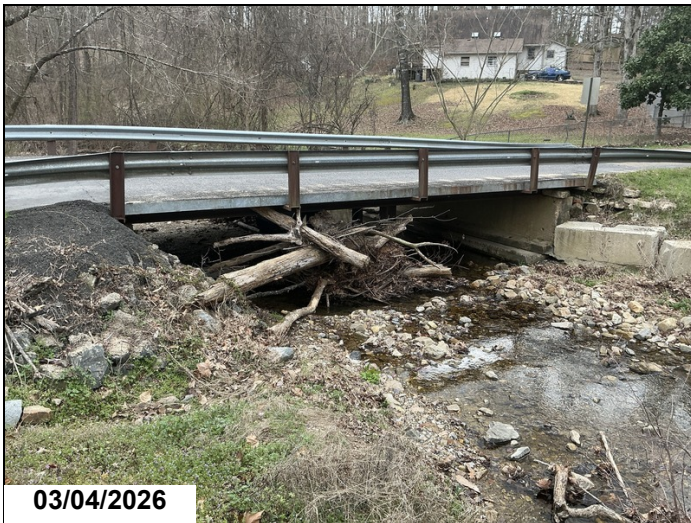
Drift and debris has accumulated at bent 2.
