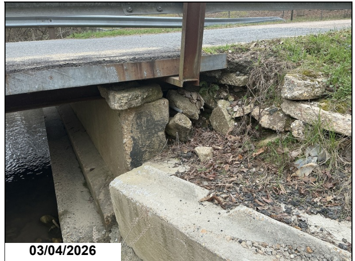
Bent 1, left side, up to 8' void behind abutment causing approach roadway to settle.
